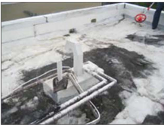
Before New Roof Installation
